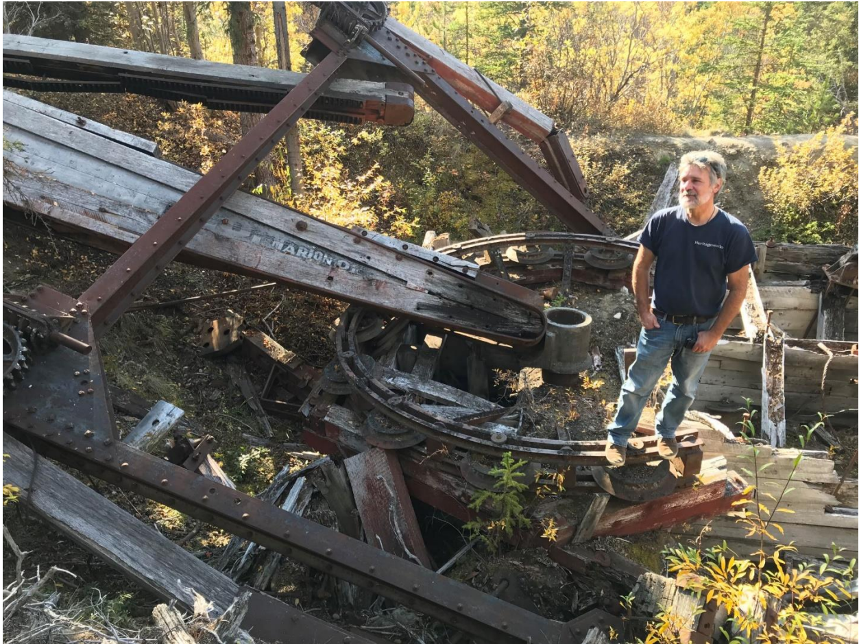
Figure 8 – The historic dredge near Atlin, September 2019.
